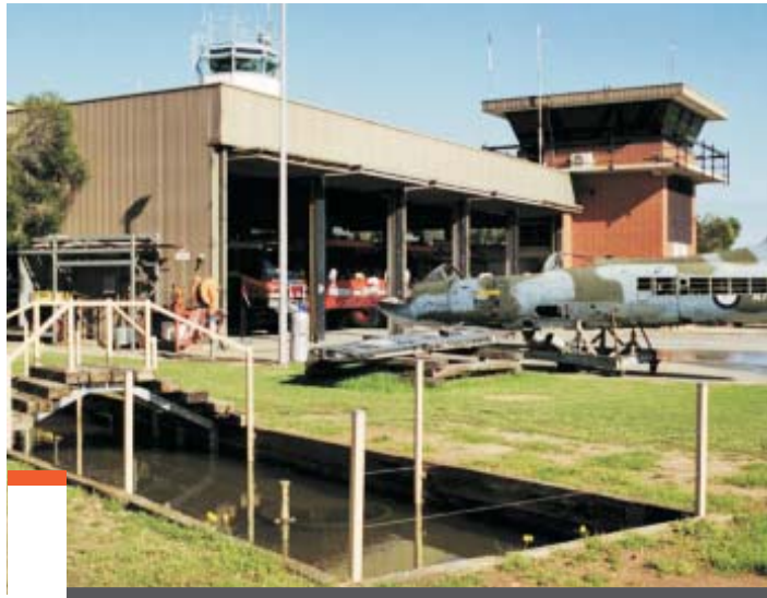
Fire station and emergency water supply at RAAF EDINBURGH, South Australia.
